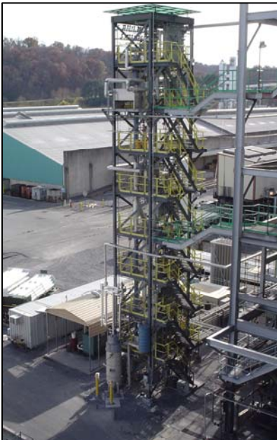
Warm-gas Cleanup - Integrated testing at Tennessee Eastman's gasification plant
